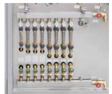
Cooling water distribution
